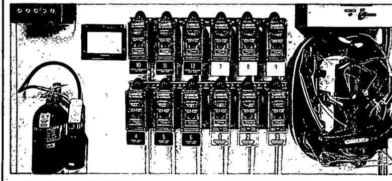
A DTC fire control station with alarms, extinguisher, carbon dioxide controls and a portable life-support unit.
