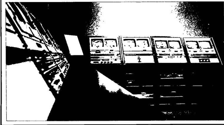
A portion of the master console in the main command post in DTC's physical security system. The monitor screens permit security guards to view what is occurring in the vault, data processing, and other secured areas. In addition, each closed-circuit camera creates a video tape record of everything in its range.
