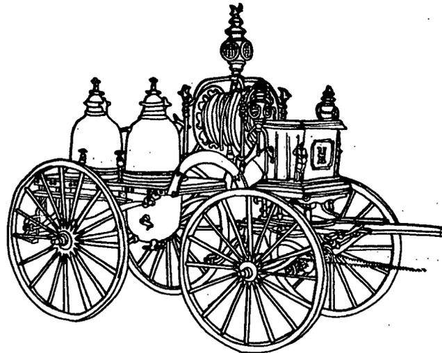
The Holloway #3 Chemical Engine consisted of two large metal soda-acid tanks and a reel of small diameter fire hose, mounted on a small hand-pulled carriage. Volunteer firemen dragged the apparatus to the fire; colored lenses on the lamp on top of the hose reel designated the name or number of the fire company.
